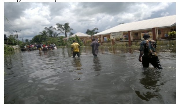
Figure 1.1: 2018 Devastating flooding in some parts of Rivers State
